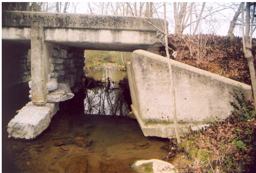
The historic bridge has a portion of the retaining wall on the southeast corner of the bridge that is in danger of collapse into the stream
