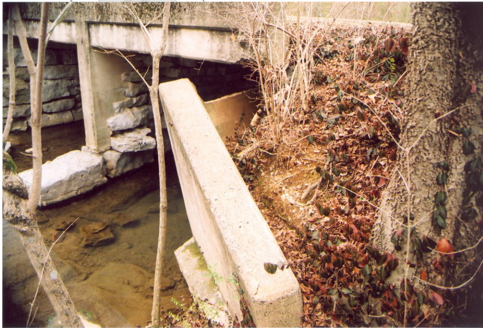
Retaining wall is leaning precariously and may soon fall into the stream
